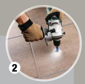
Once the drill bit is inside the material, make sure the angle between the drill bit and the material reaches gradually 90°.
